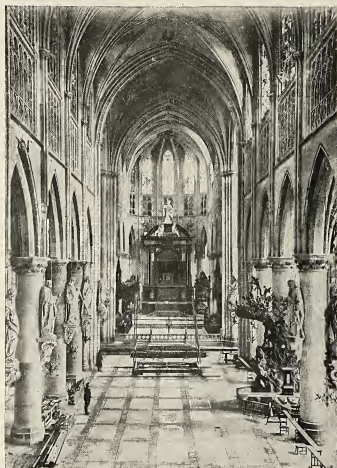
Malines. Interior of the Cathedral after the bombardment in August 1914
